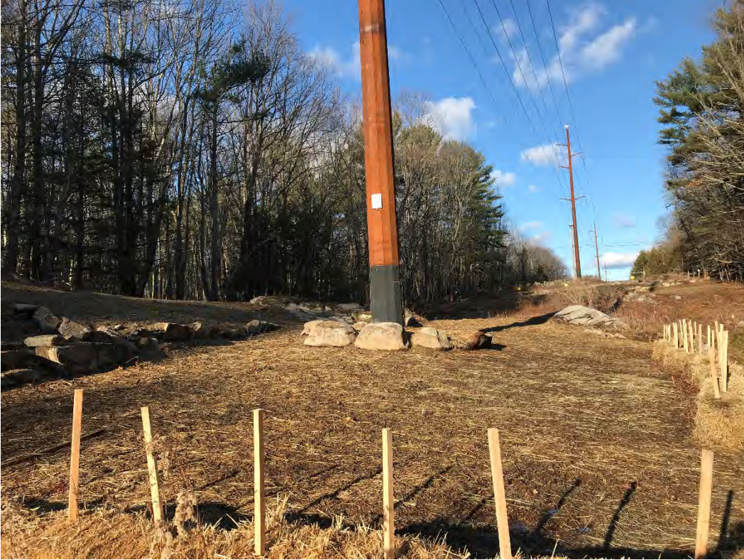
Fig 5: Str. 89 work area. Viewing northwest. (12-26-20)
