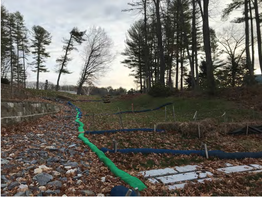
Fig 9: Slope above the manhole at Gundalow Landing/east side of the bay. Viewing east. (12-30-20)
