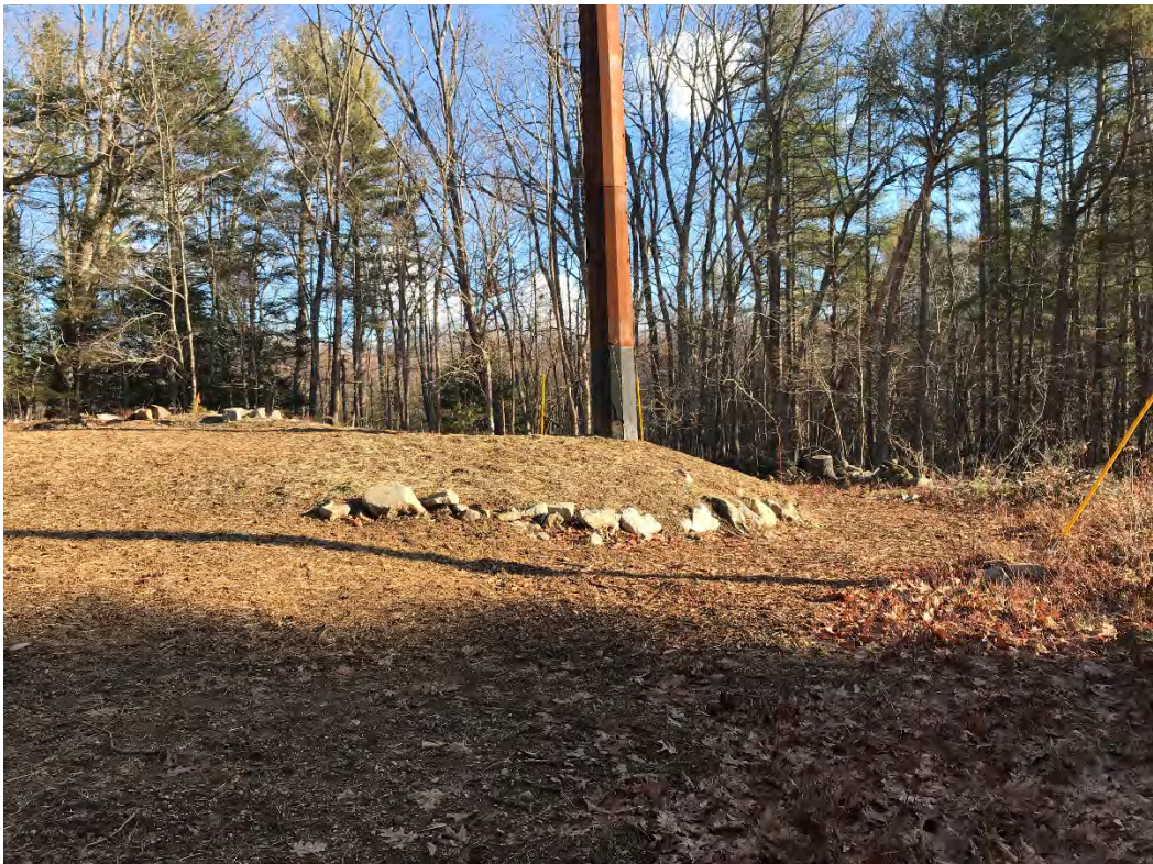
Fig 6: Str. 90 work area. Viewing northeast. (12-26-20)
